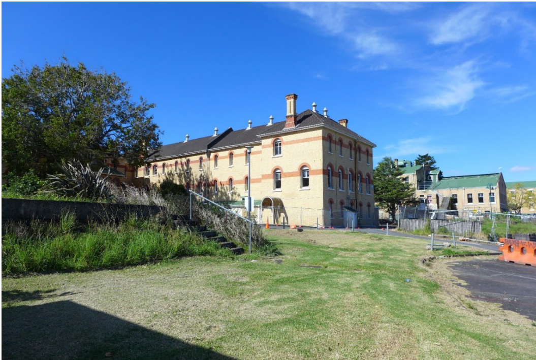
fig. 1 former asylum building, 1 carrington road.
